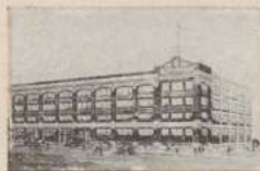
Cincinnati, O. 4 stories 236 x 159—150,096 square feet floor space
