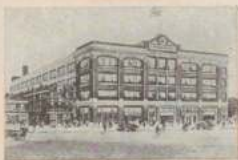
Indianapolis, Ind. 4 stories 250 x 142—142,000 square feet floor space
