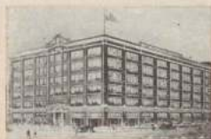
Chicago, Ill. 6 stories 592 x 164—582,528 square feet floor space
