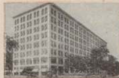
Detroit, Mich. 8 stories 320 x 97—248,320 square feet floor space
