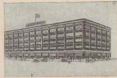
Milwaukee, Wis. 5 stories 300 x 120—180,000 square feet floor space
