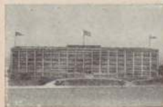
Des Moines, Ia. 5 stories 453 x 120—271,800 square feet floor space
