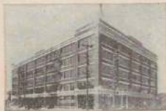
Los Angeles, Cal. 5 stories 200 x 150—150,000 square feet floor space
